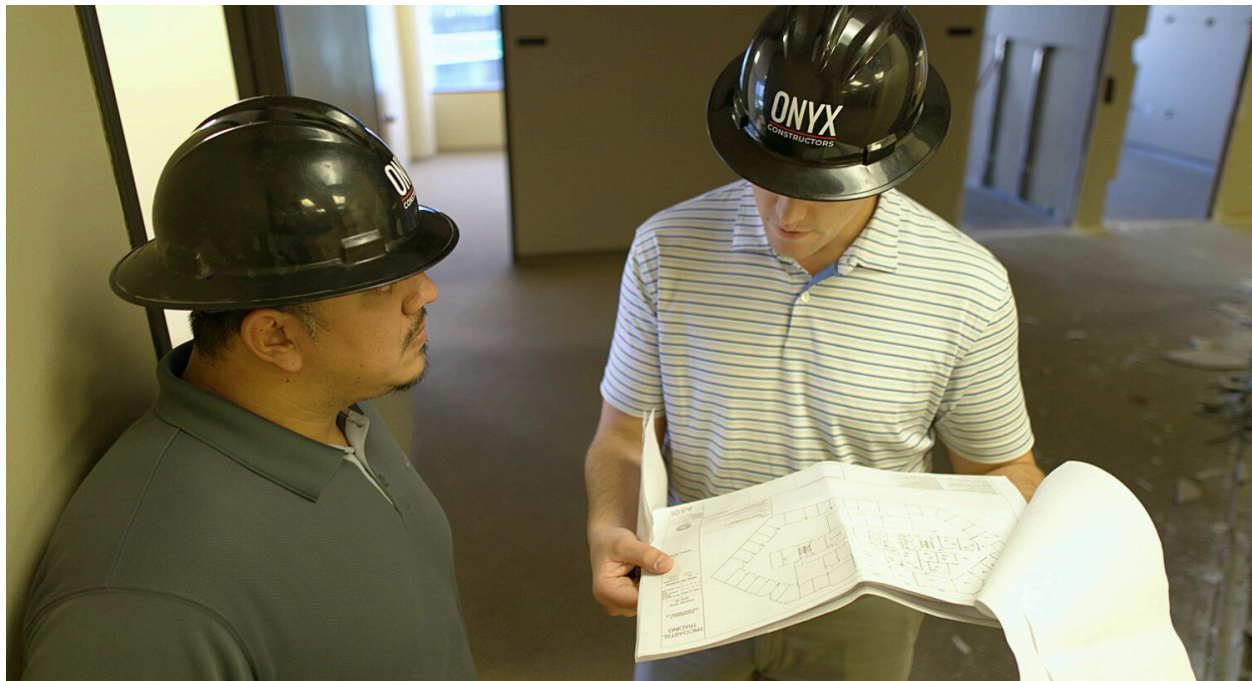
Plans and specifications are constantly monitored to ensure the team is executing as required.
