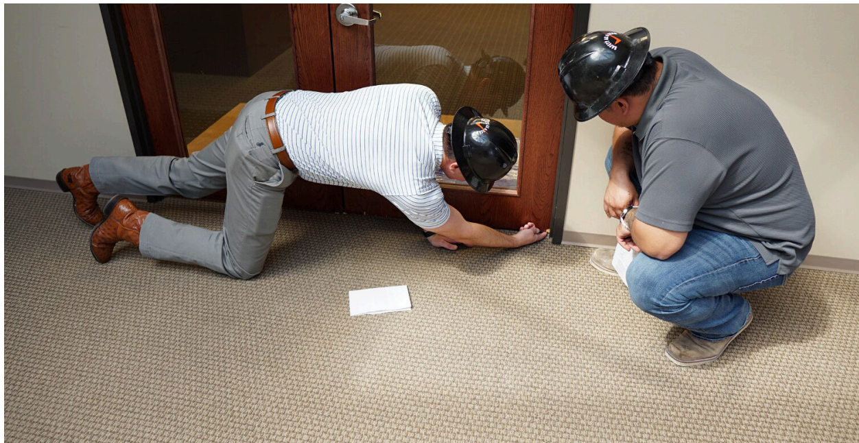
Quality control procedures are in-place from the beginning through completing the final punch list.
